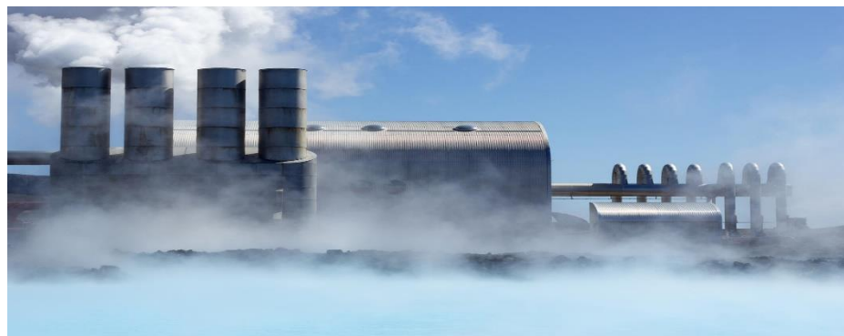
The Svartsengi geothermal power plant near Grindavík, Iceland Daniel Snaer Ragnarsson/iStock
