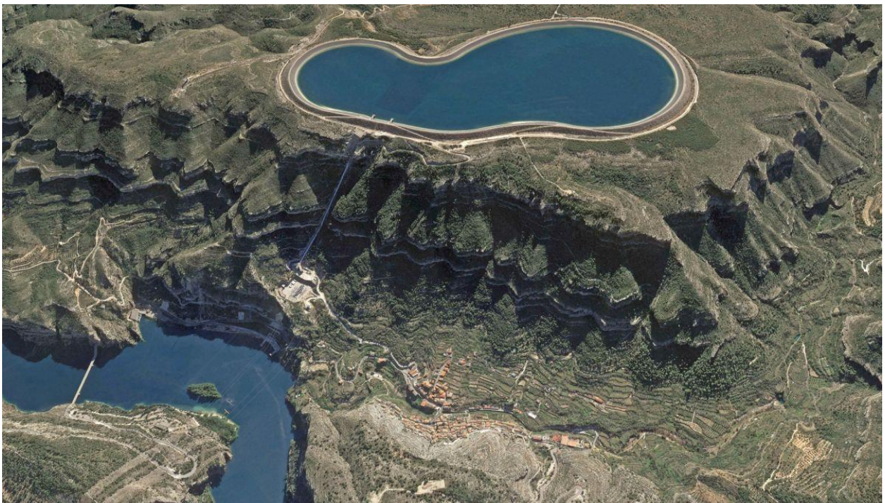
A pumped hydro energy storage plant in Spain. (Image credit: Burakyalcin/Shutterstock.com)
