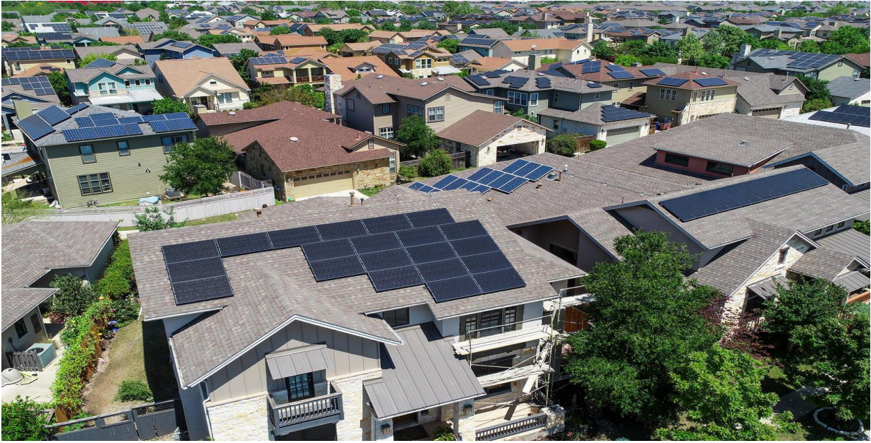
Solar panels on the rooftops of East Austin, Texas
